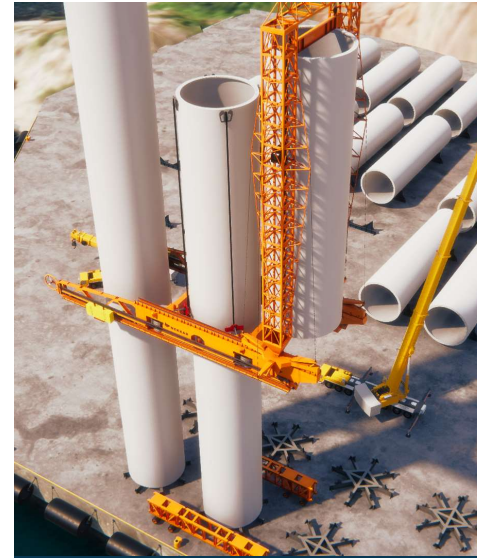
Installation of tower sections for bottom fixed offshore
