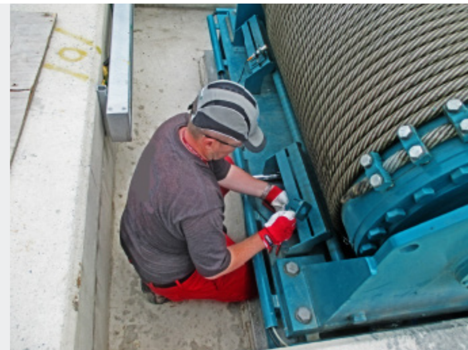
Montage of Syncrolift parts
